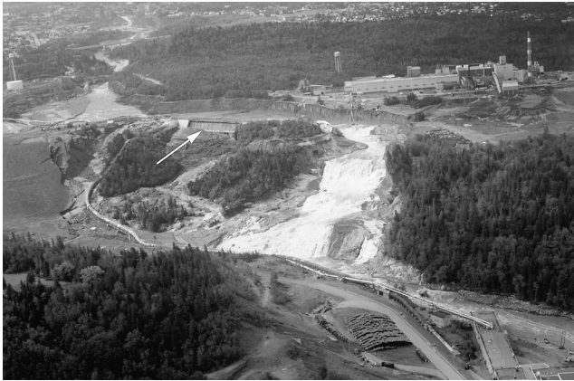
FIGURE 11. Post-flood view of the Chute-à-Besy dam, taken on July 26, 1996. The entire flow of the river has been diverted through the breach, as discussed in the text. The intact, but non-functional dam is marked by an arrow.
