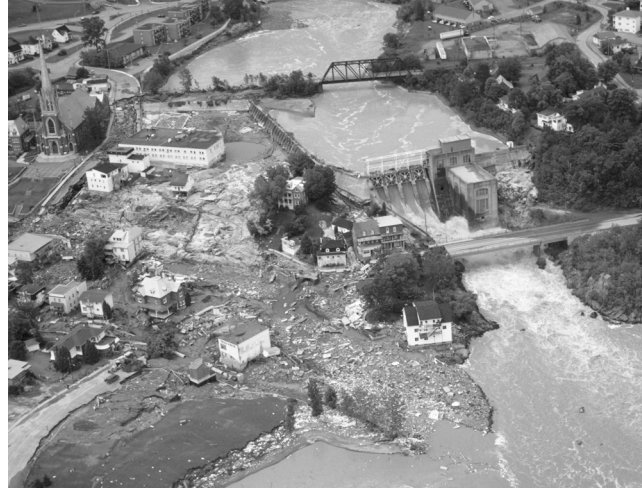
FIGURE 12. Post-flood view of the Chicoutimi dam located in downtown Chicoutimi, taken on July 26, 1996. During the flood, floodwaters overtopped the buttressed concrete wing-wall of the dam that extends to the left of the control structure in the photograph, and flowed rapidly through the residential-commercial area situated immediately down slope. Along the flow path, overburden and road beds were scoured in places to bedrock, and buildings were washed away or damaged. A bar composed of bed materials extends into the pre-flood channel (bottom centre right of photograph), where the flood flow re-entered the river .
