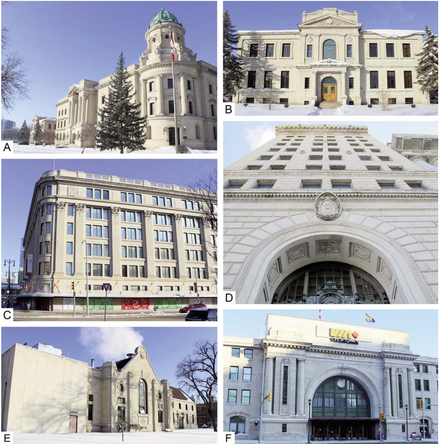
Figure 24. Older buildings using Tyndall Stone, Winnipeg. A. Law Courts (1916). Beaux Arts style. B. Land Titles Building (1904). Neo-classical style. C. Hudson's Bay Company Building (1926). Neo-classical style. D. Hamilton Building (1918). Chicago School style. E. Manitoba Power House (1915). F. Union Station (1911). Neo-classical style.
