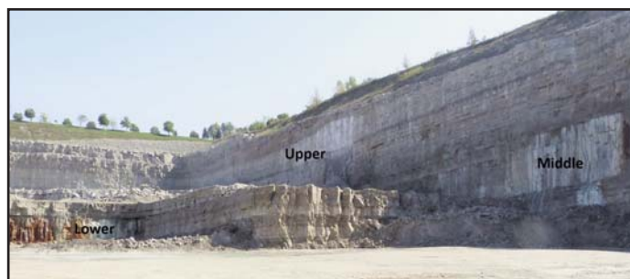
Figure 17. Inflow of sulphur water along bedding plane partings in the Lucas Formation on the southern face of the McGregor Quarry. Inactive zones are marked by white residue immediately below the bedding plane. The red staining on the lower bench marks an active inflow with a rotten egg smell, indicative of the presence of sulphur-oxidizing bacteria. Exposed bedrock thickness is approximately 40 m. Photograph taken October 18, 2013.
