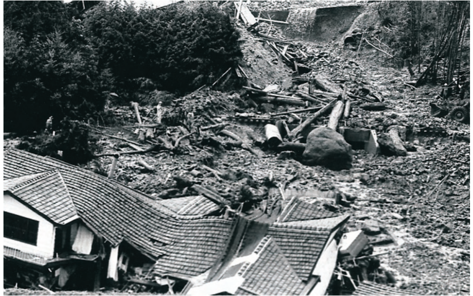
Figure 10. Aftermath of a debris flow that swept down Alberta Creek and through the community of Lions Bay in February 1983, killing two people. Source: Vancouver Sun.
