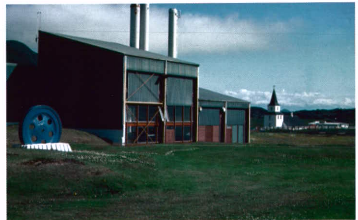
Figure 8 (at left) Photo/diagram schematic through one of the Vestmannaeyjar heating units. Figure 9 (above) The geothermal water distribution plant in central Vestmannaeyjar.
