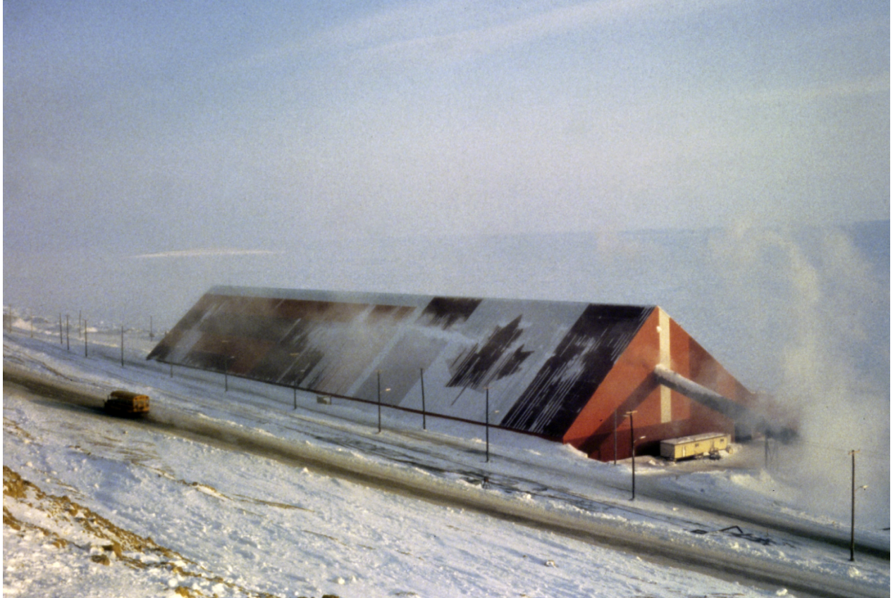
Figure 5. Ore shed, Polaris mine, ca. 1990. Photo: LCI. Source: NWT Archives/Northwest Territories. Dept. of Public Works and Services Fonds, G-1995-001: 1517.
