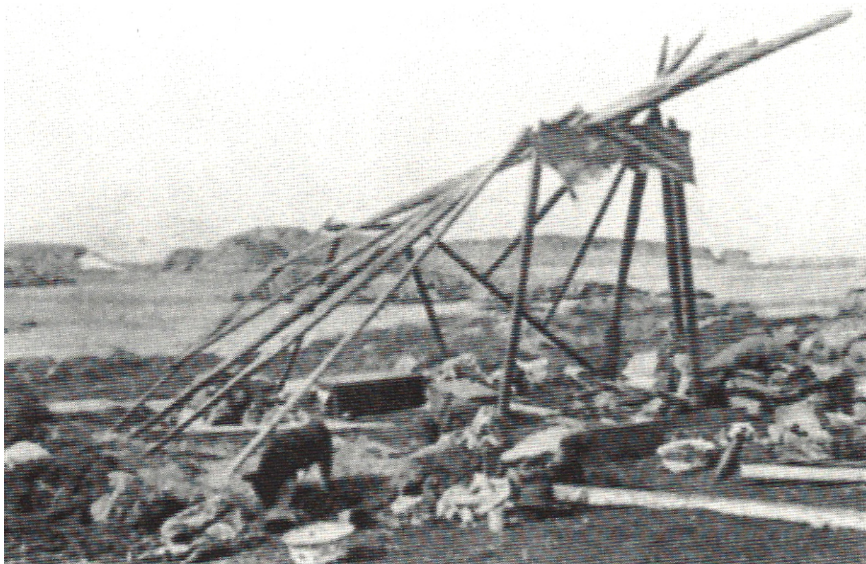
Figure 7. The structural frame of an erqulik , or double-arch tent. Source: Birket-Smith (1924: fig. 119).
