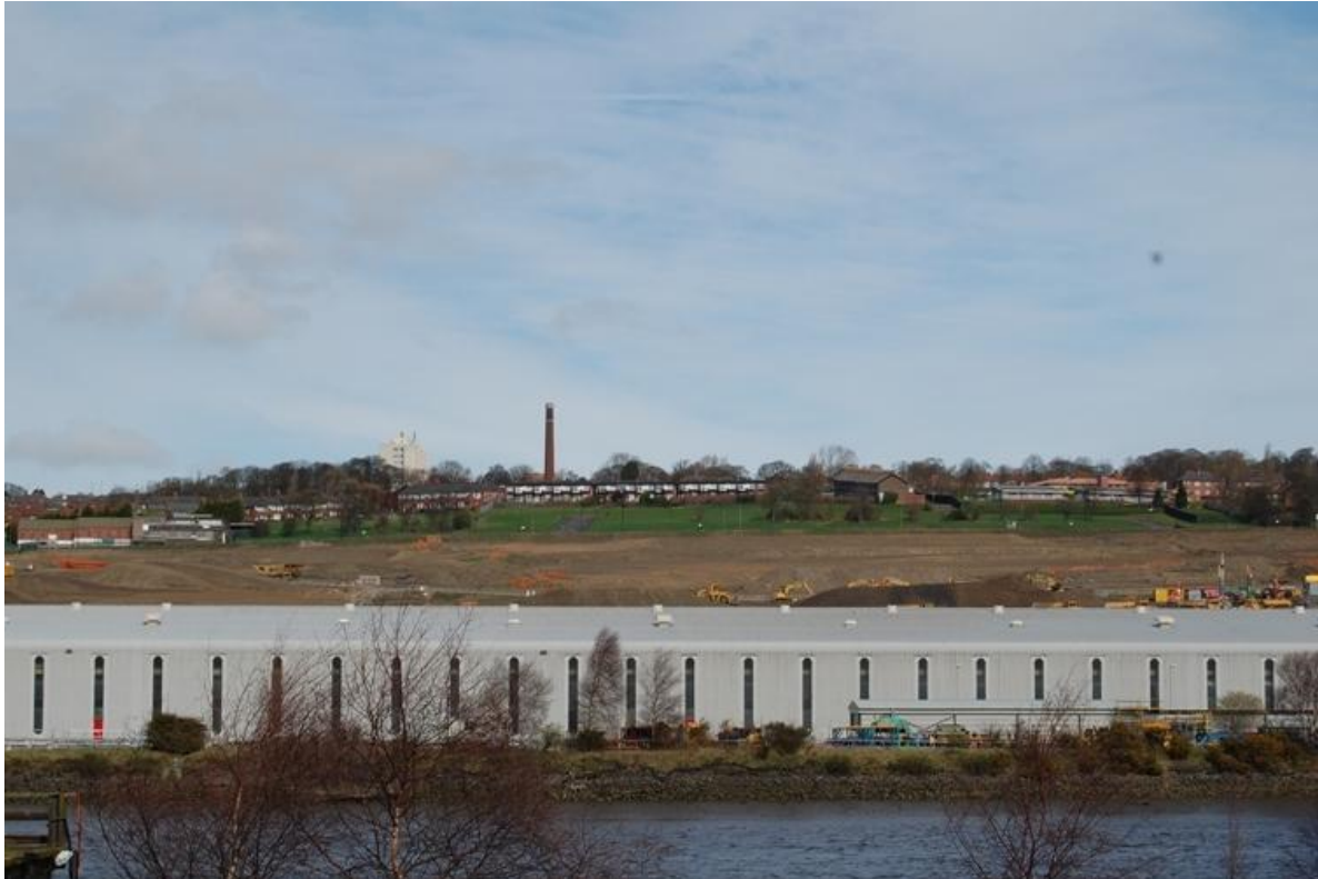
Figure 14 The Armstrong works with Scotswood beyond
