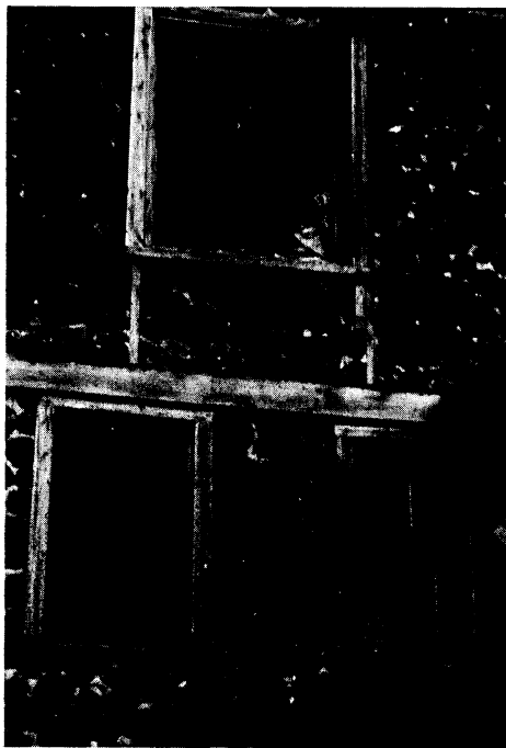
Photo 3 Stove-wood (or log-but) construction. A barn north of Saint-Jovite.
