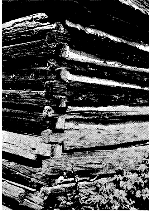
Photo 5 Squared - log construction with simple square lapped cornering and wide, chinked spaces between logs. Barn near Lac Matilda in Arundel Township.
