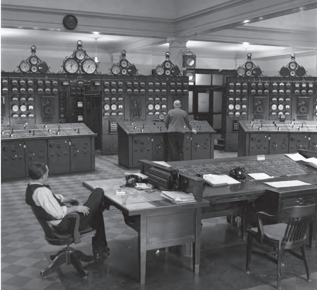
Figure 2. Control room of the Queenston hydro-electric plant. Library and Archives Canada 1971-271 NPC.
