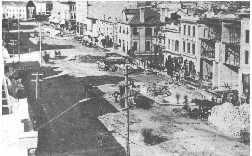
FIGURE 6. Construction on Main Street, 1882.
