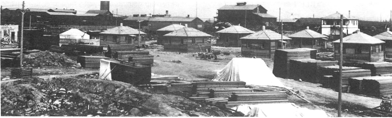
FIGURE 3. Company cottages being built for H.B.M.&S. staff and employees, c. 1929.
