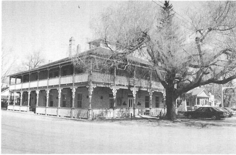
FIGURE 3. The Little Inn — restored hotel in Bayfield.
