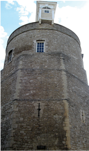
Figure 1. The Bell Tower, Tower of London, Exterior
