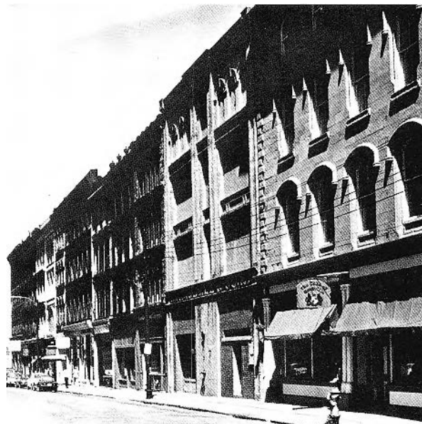
FIGURE 4. William Thomas and Sons and others, Buildings on north side of Granville Street, Halifax, 1859 ff (Photo: Harold Kalman).
