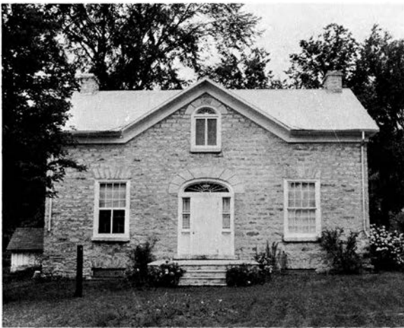
FIGURE 18. House on the Mississippi near Lanark. (Photo: Shackleton)
