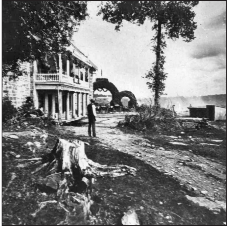
Thomas Barnett's Niagara Falls Museum at left, with mist from the falls visible in the background. (Niagara Falls Public Library)
