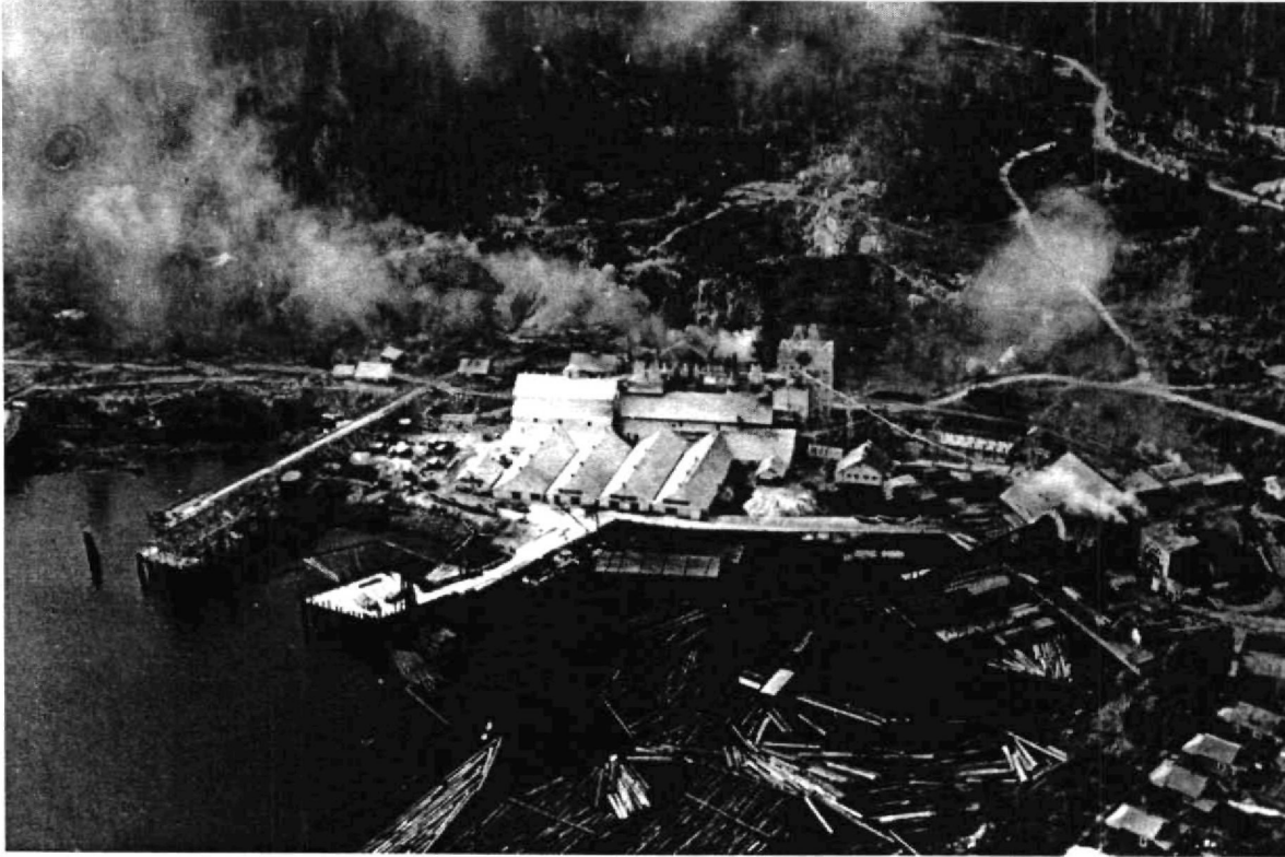
Figure 4. The Pacific Lime Company operations at Blubber Bay. On the far left of the picture is the bunkhouse used by Chinese workers; in the lower right hand corner are the company houses used by white workers. Behind the main lime processing operation (centre) is the “glory hole” — the massive open pit lime mine. (BCARS, AVRU, #11631 A-4516)
