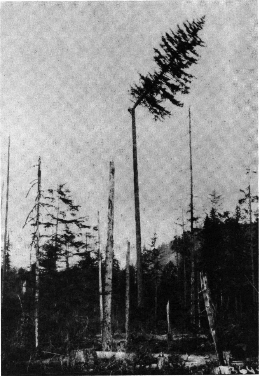
High rigger topping spar tree. Photograph #73645, B.C. Archives and Records Service.
