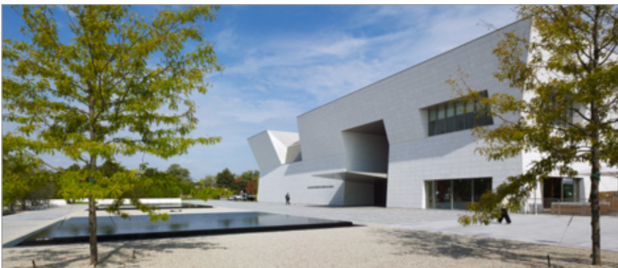
FIG. 1. VIEW OF THE SOUTH CORNER OF THE AGA KHAN MUSEUM (AKM), DESIGNED BY FUMIHIKO MAKI, WITH ITS PUBLIC ENTRANCE MARKED WITH A THIN METALLIC CANOPY, FACING THE PLAZA LINKING IT TO THE ISMAILI CENTRE DESIGNED BY CHARLES CORREA (NOT VISIBLE IN THIS IMAGE). | COURTESY OF THE AGA KHAN MUSEUM, PHOTOGRAPHER TOM ARBAN.
