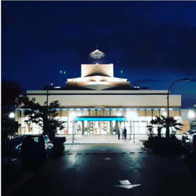
FIG. 26. AT NIGHT, THE NORTH ELEVATION OF THE KHALSA DIWAN SOCIETY VANCOUVER GURDWARA, 8000 ROSS STREET [KHALSA DIWAN ROAD], VANCOUVER, SHOWING THE STEEL AND GLASS PAVILION NOW FRAMING THE MAIN ENTRANCE: [HTTPS://WWW.FACEBOOK.COM/KDSROSS/PHOTOS/4854923237868748]. | THE KHALSA DIWAN SOCIETY VANCOUVER.
