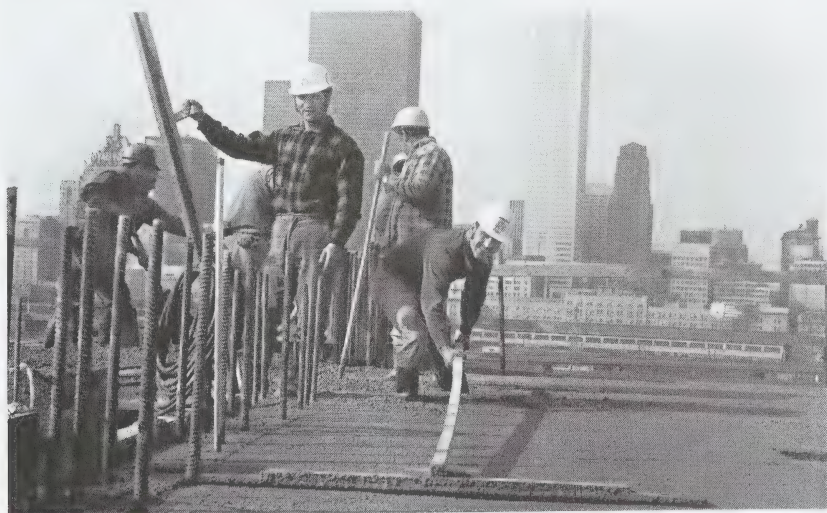
Fig. 4. Fourteenth floor of Harbour Castle Hotel, waterfront, 1973. ( Not Paved with Gold , 34-35.)
