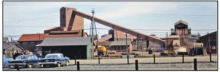
Figure 20. No. 3 mine deck head and float-sink mill and infrastructure added during mine expansion and modernization in the late 1950s. Source: Memorial University of Newfoundland–Digital Archives Initiative.
