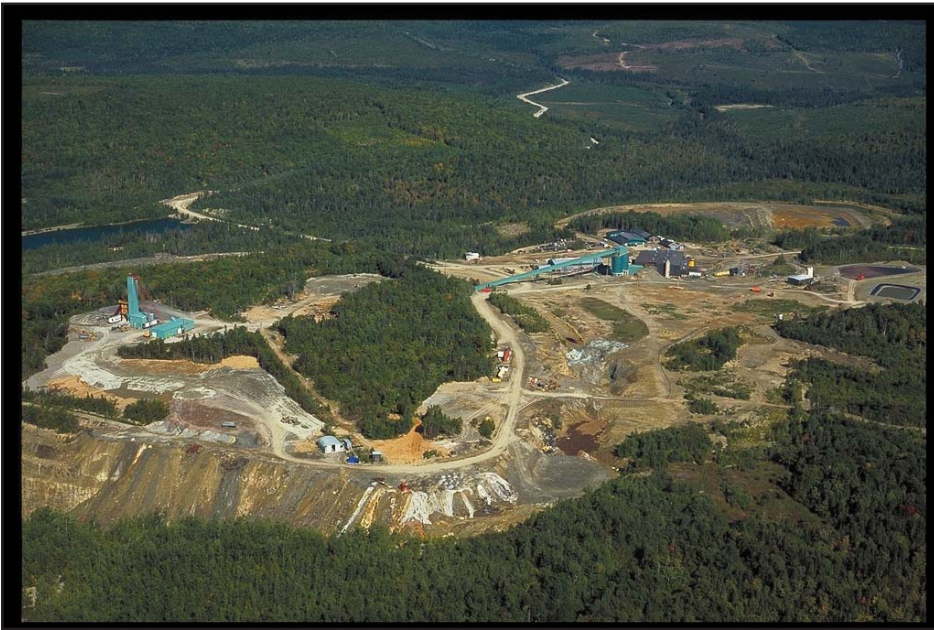
Figure 3. Aerial view of the Caribou Mine (circa 1997).
