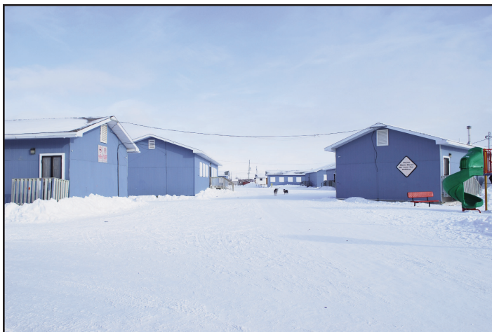
Figure 2. View of the portables at J.R. Nakogee Elementary School.
