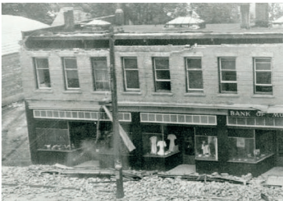
Figure 8. Damage to the Bank of Montreal building in Port Alberni, BC, resulting from the M 7.3 earthquake of 1946.
