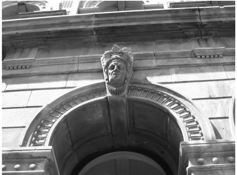
Figure 8. Sandstone from the Caledonia Quarry in eastern New Brunswick was used to build the 'Old Post Office' in Saint John, ca. 1877-80.
