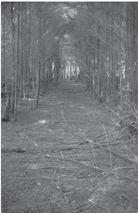
Figure 5. An abandoned corduroy road constructed in the early 1900s across peatland on Graham Island, Queen Charlotte Islands, British Columbia.
