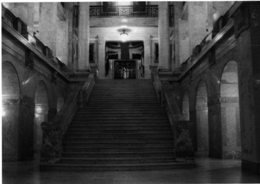
Figure 10 Grand staircase leading to the Legislative Assembly Chamber on the first floor of the Legislature. The floor of the Rotunda, the steps and balustrade of the staircase are in Quebec marble as is the paneling of the colonnade (Provincial Archives of Alberta PA 43/12).
