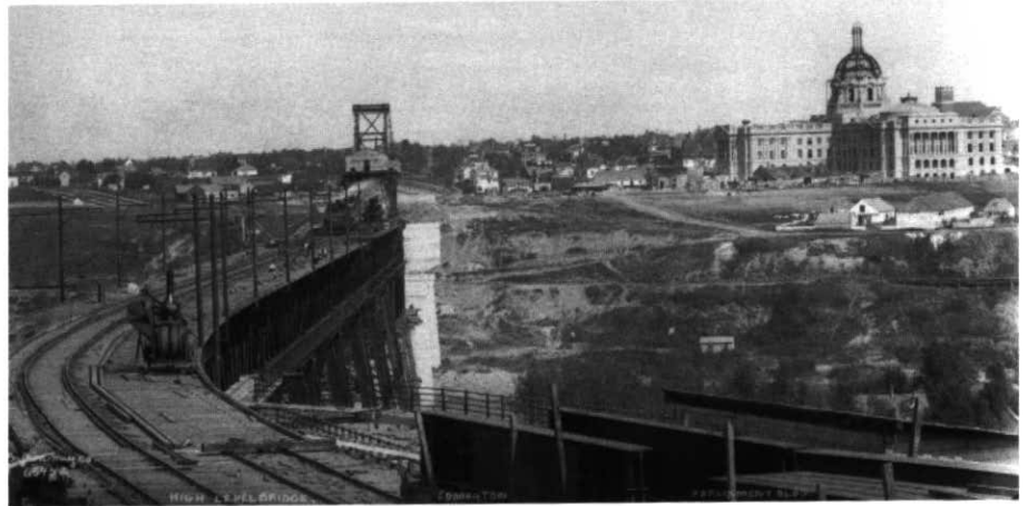
Figure 5 The Legislature from the south bank of the North Saskatchewan River. The High Level Bridge and the dome of the Legislature are under construction. Fort Edmonton still stands on the crest of the north bank of the river overlooking the Edmonton Yukon and Pacific Railway (Glenbow Archives NC663752).
