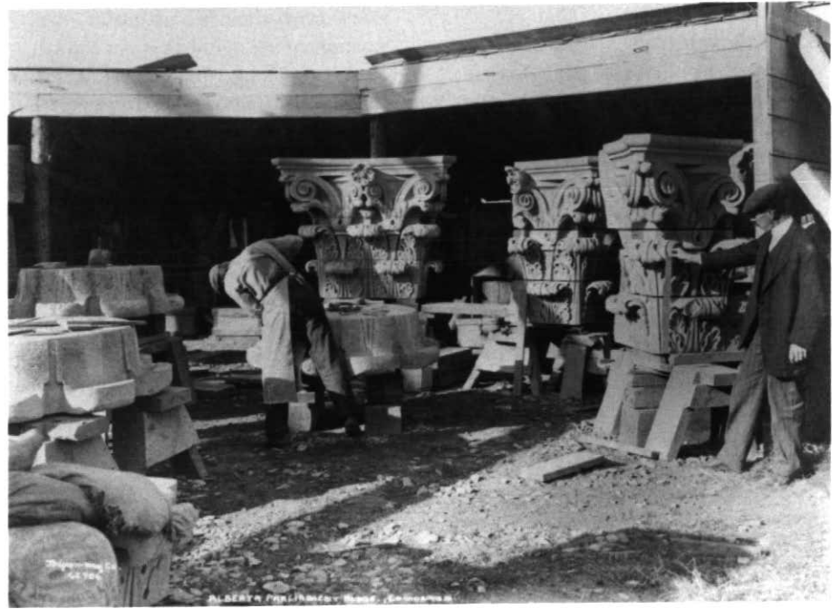
Figure 8 The carving of composite Corinthian capitals for columns and pilasters in the portico of the north, main entrance of the Legislature. Carved Alberta roses (the provincial flower) surmount oeil de boeuf and acanthus volutes (Glenbow Archives, NA 1042–10).
