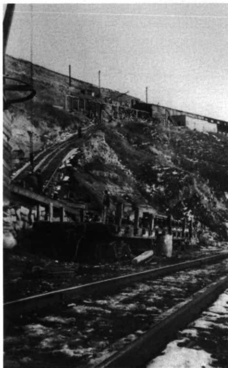
Figure 7 The Glenbow Quarry, 25 km west of Calgary on a siding from the Canadian Pacific Railway in the Bow River valley. Stone, quarried towards the crest of the valley was cut and trimmed in the shops below before being carried by the inclined tramway to loading facilities on the railway spur (Glenbow Archives, NA1025-1).
