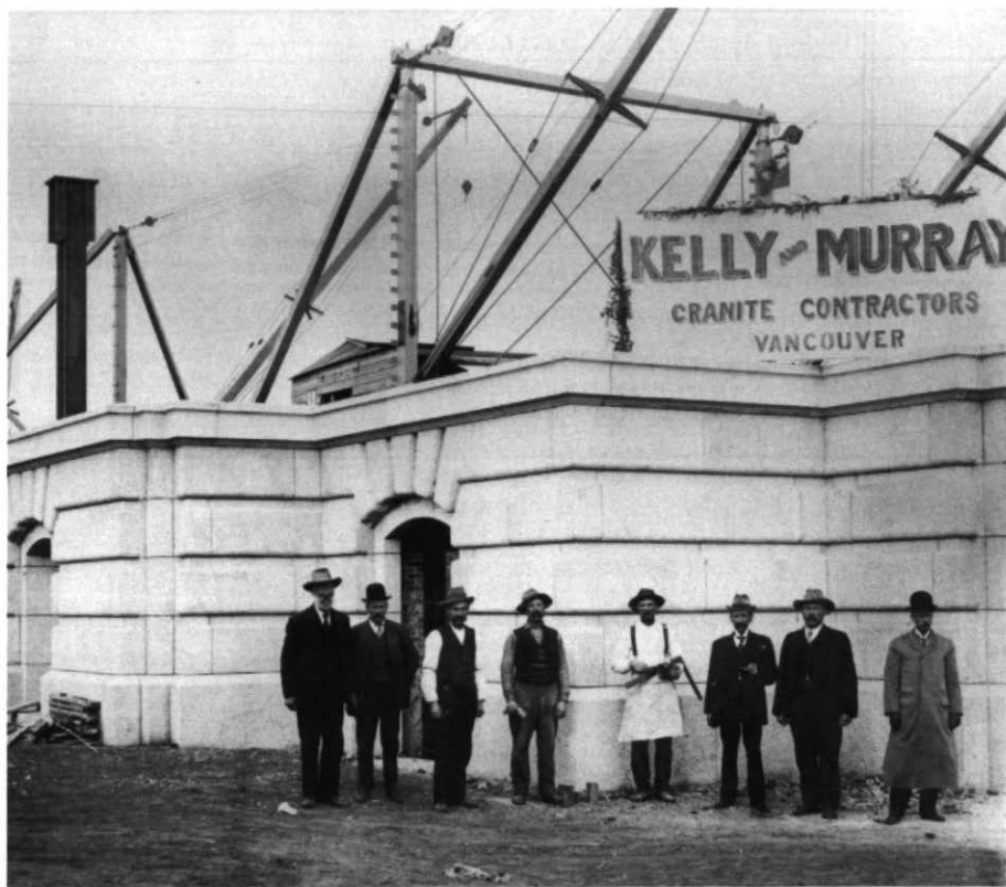
Figure 3 The recently completed granite walls of the Legislature support the contractor's sign in 1909. Allan Jeffers, the architect stands with building superintendent, John Gillespie and unidentified coworkers to his right. Steam-powered cranes in the background were used for placing stone. The doorway behind the coworkers reveals the brick backing of the stone (Glenbow Archives, NA 10428).
