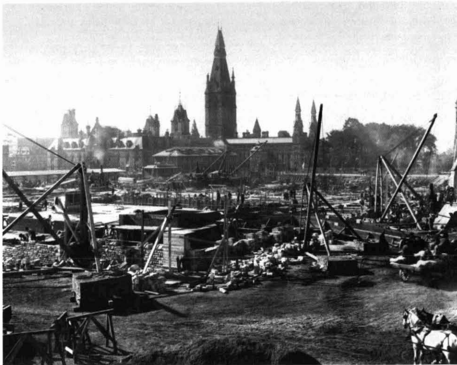
Figure 4 View looking southwest showing the early stages of the reconstruction of the Centre Block. Beyond the construction on the left is the stone cutting shed and to the right the architect's offices. The West Block is in the background. Photo taken 26 September 1916. National Archives of Canada C6361.
