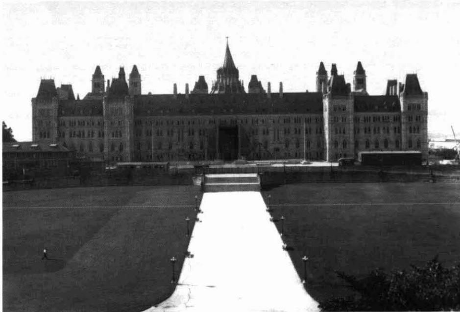
Figure 12 The nearly completed Centre Block, in 1919. Construction of the Peace Tower had not been started at this time. The stone masons' shed and the architect's site office can be seen on the left in front of the building. W.J. Topley, National Archives of Canada PA 12925.
