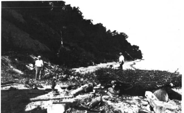
Figure 7 Early attempts at remedial work: "Mississippi mats" constructed by laying brushwood, mostly willow, on a wooden frame, being placed around the intake for the Scarborough Waterworks (Fig. 3) in the mid 1930's (from the collection of A.P. Coleman)
