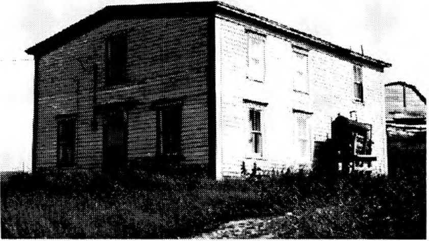
Fig. 9 - Allan McArthur's house, Upper Ferry, before renovations.
