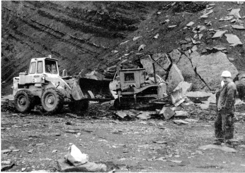
Figure 1. A bulldozer and payloader prepare to remove the track-bearing slabs (on right) from the bottom of the Joggins cliff.
