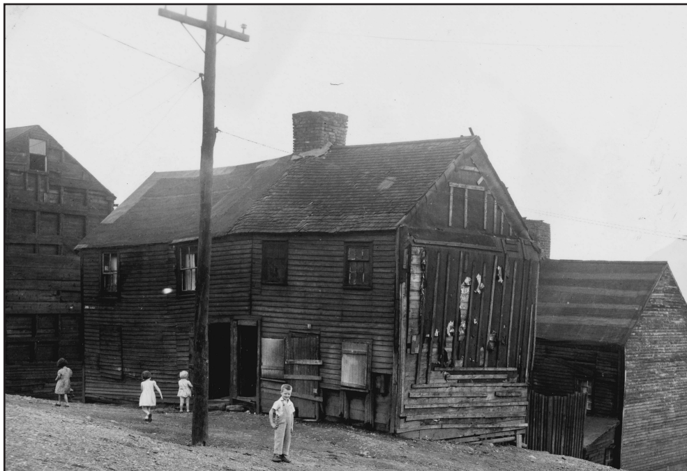
Source: Photo 11-02-036, City of St. John's Archive.
