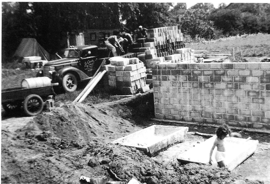
Figure 6: More blocks being delivered by the J. Cooke, Concrete and Blocks Company of Aldershot to complete the foundation, as Glenda Hall, their youngest daughter, wanders by the site, June
