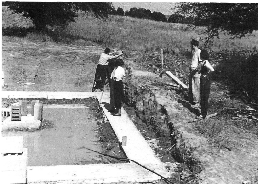
Figure 5: The footings being poured for the basement, June 1949.
