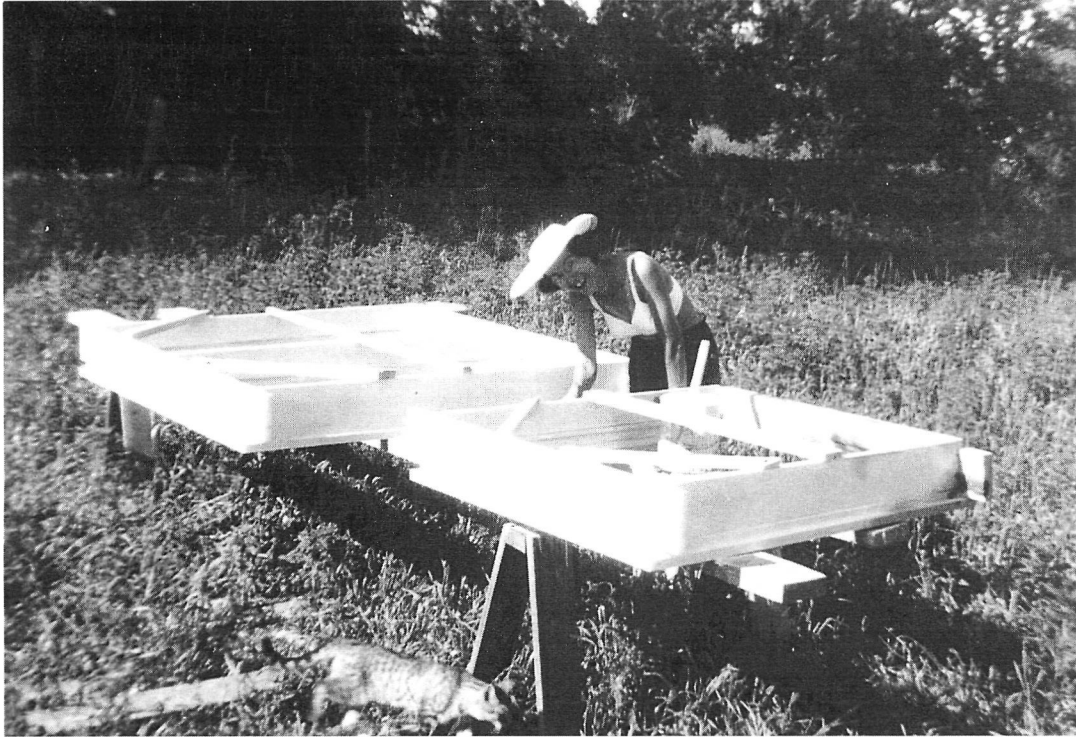
Figure 7: Mrs. Hall painting the windows that were installed once the walls were complete, June 1949.
