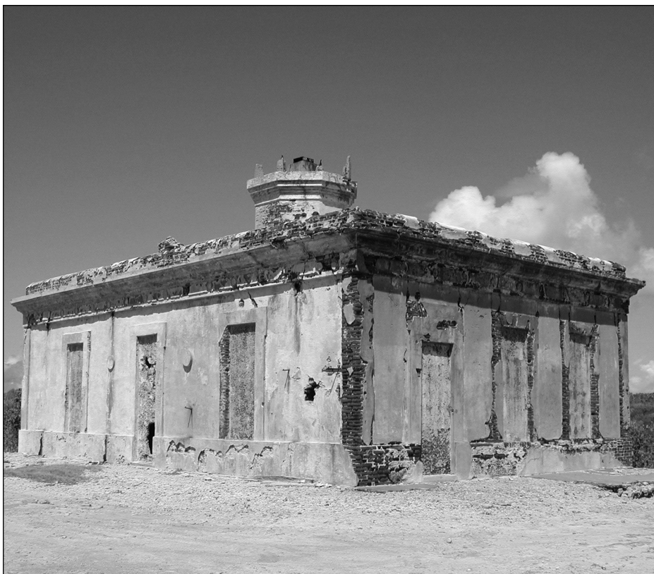
Historic lighthouse, Vieques (Puerto Rico).
