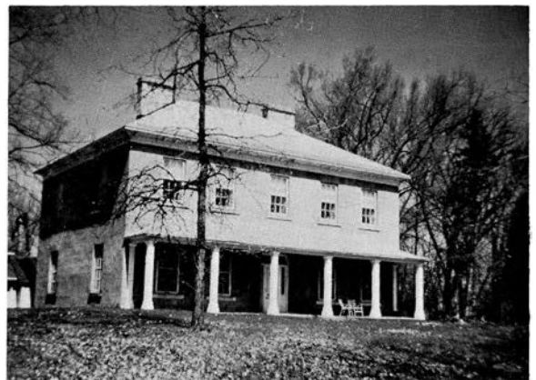
FIGURE 5. The Haggart-Shortt house, Perth, built 1837 for John Haggart, a Scottish miller. (Photo: Jean Norry )
