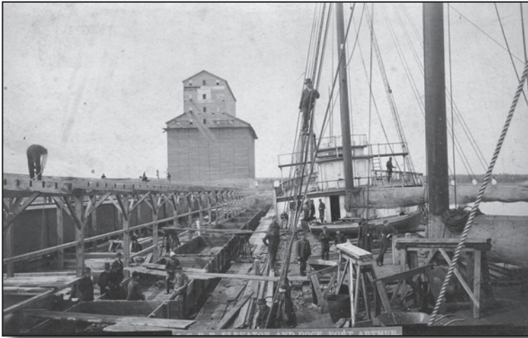
Canadian Pacific Railway's first Lakehead grain elevator and dock under construction in 1883. J.G. King leased it in 1891. Thunder Bay Historical Museum Society 973.27.43.
