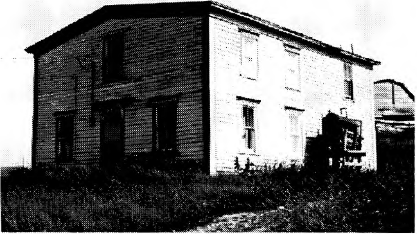
Fig. 9 - Allan McArthur's house, Upper Ferry, before renovations.
