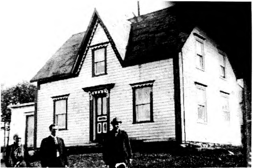
Fig. 10 - Allan McArthur's house, Upper Ferry, after renovations.
