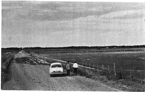
Photo 3 Overflow from flooded field still drains onto the public roads.
