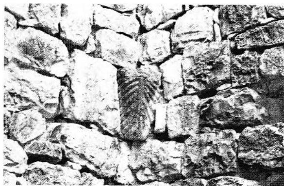
FIGURE 31. As in Fig. 30. Detail. Corbel (Photo: Author).
