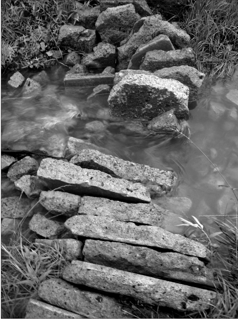
Fig. 7 Demolished grey infrastructure is inverted and reused as stormwater detention weirs. Photo by author.
