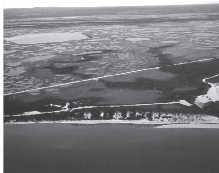
Figure 7. Oblique aerial photograph looking north of Hwy. 138 between Sept-Îles and Havre St. Pierre, Quebec. The earlier abandoned highway with several large failures exposing the underlying glaciodeltaic sand deposits is located next to the Gulf of St. Lawrence. The new highway is farther north with small washouts exposing sand along it.
