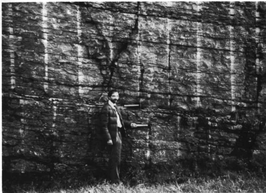
Figure 11 Offset boreholes exposed along the St. Laurent exit ramp off Autoroute 50 in Hull, Quebec. The average direction of offset is 070^\circ , which coincides well with regional S_{Hmax} orientations determined from hydraulic fractures, breakouts and earthquake focal mechanisms. Details are given by Wallach et al. (1995).
