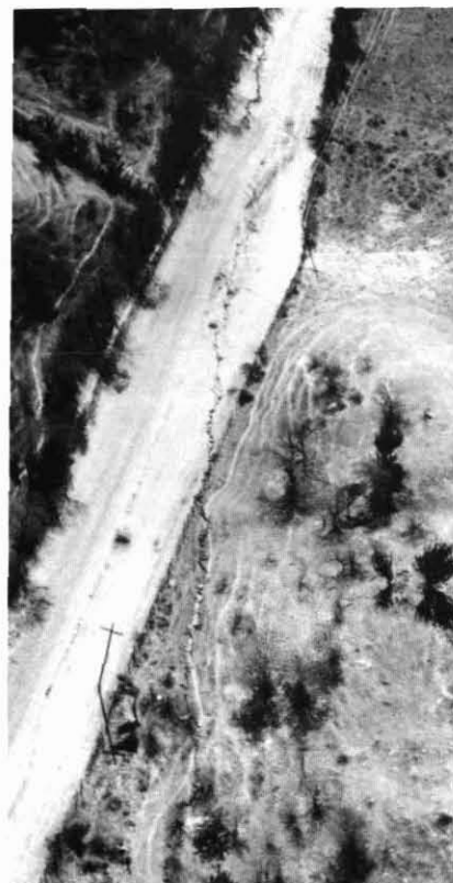
Figure 3 Faultbreak, easily visible as it crosses a dirt road, note the right-stepping en echelon pattern, which was generally observed.
