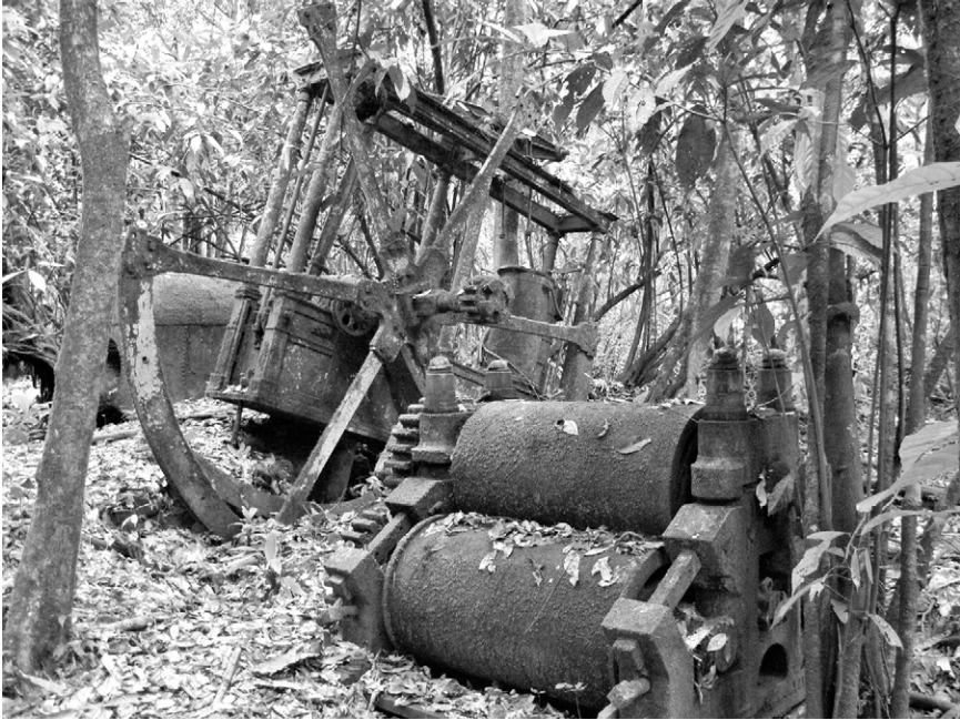
Figure 4. Machine de Watt de l'Habitation Constance, Bas Approuague, Guyane. © Apolline Fluck
