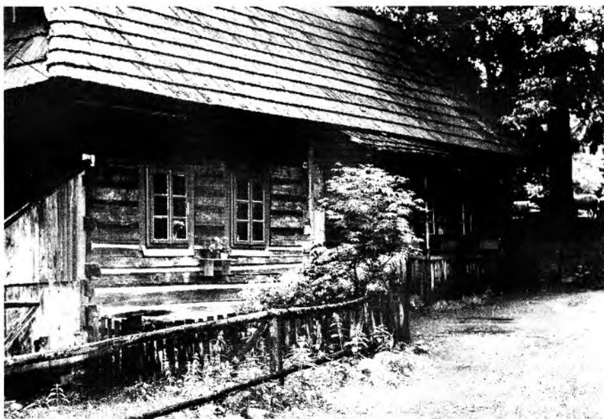
1. Regional style log construction, Villa "Tea." Photograph by T. Cooley.
