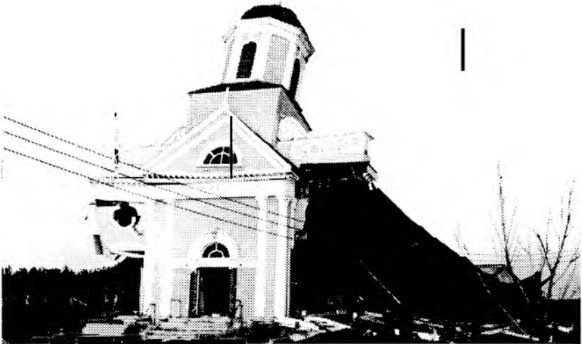
Fig. 6 - St. Anne's Church being torn down, 1982, Searston.
