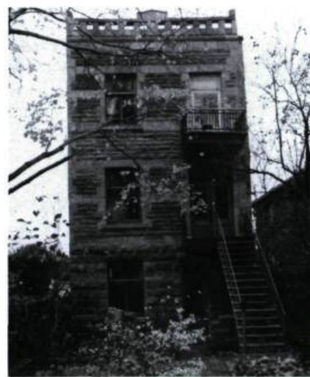
Triplex, 1229-1231, Mont-Royal (Asselin & Perron, arch.; 1905). Photo: P.-R. Bisson et Ass.
